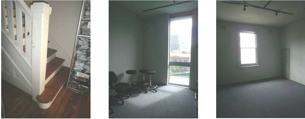
Figure 15 Photographs of the remaining original stair and finishes within two of the rooms in 161-165 Brougham Street. Photographs courtesy City of Sydney.
